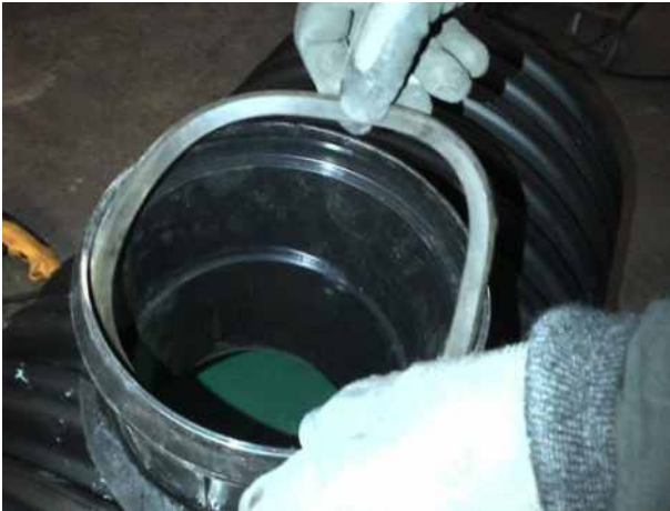
Only for connections with PVC pipes: position the EN 1401 gasket into the fitting's lodgings
