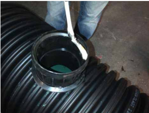
Lubrication of gasket EN 1401 for connection to PVC pipes
