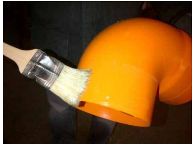
Lubrication of pipe/fitting before connection
