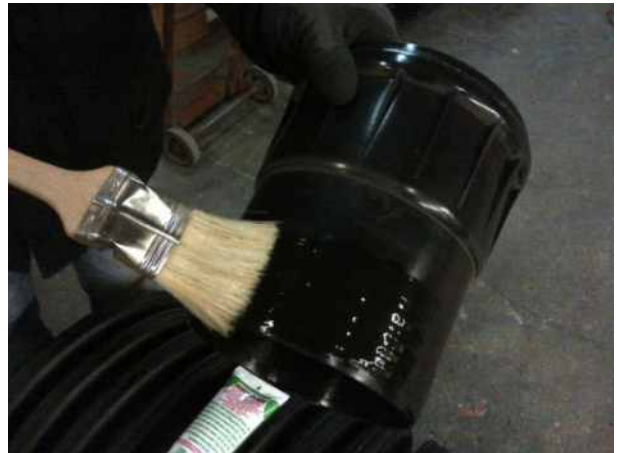
Lubricate the external part of the special fitting
