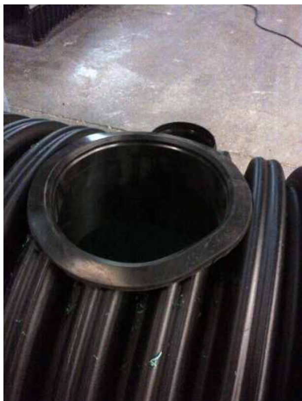
Position the seal in the hole
