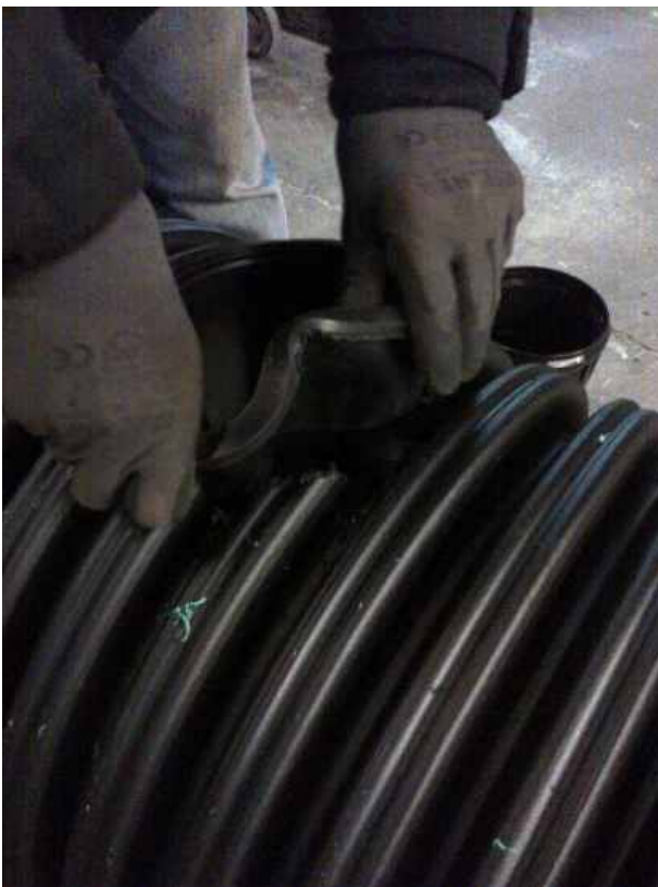
Position the seal in the hole
