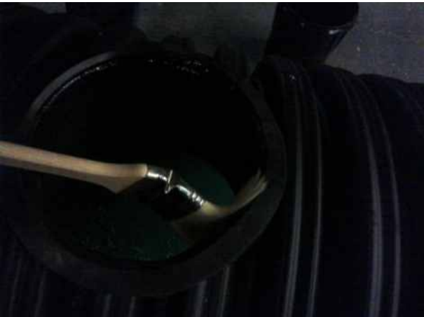
Lubricate internal part of seal
