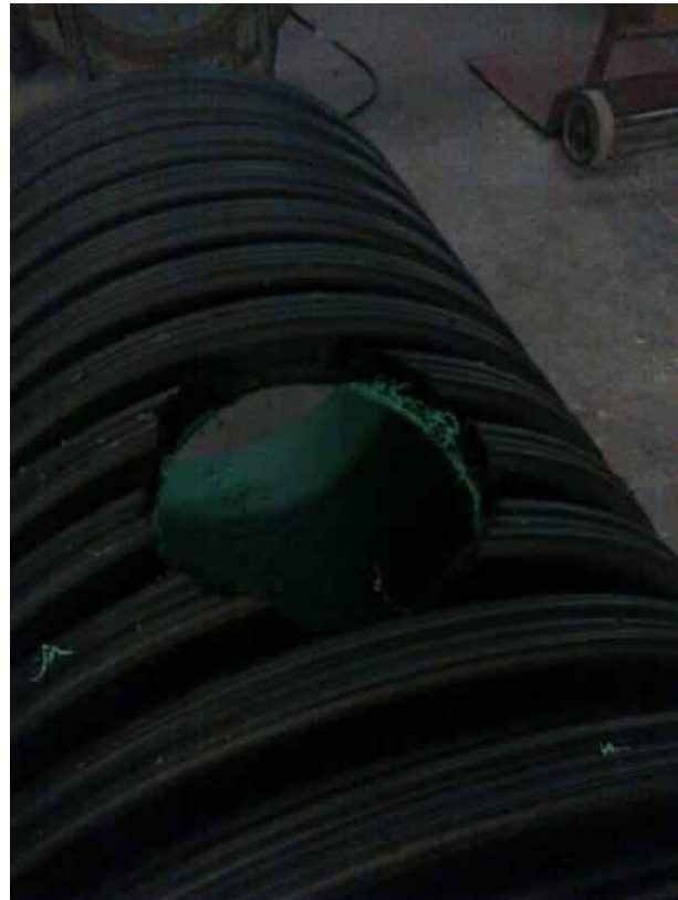
Hole as it is after drilling operation
